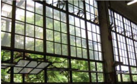
Figure 76. Steel frame windows in South Facade (Author,2010).
