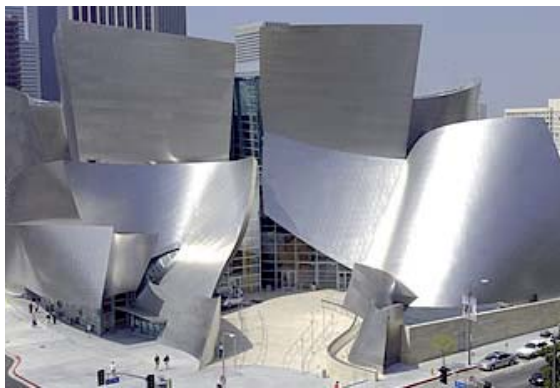
FIG 4.7_ Exterior stainless steel cladding
