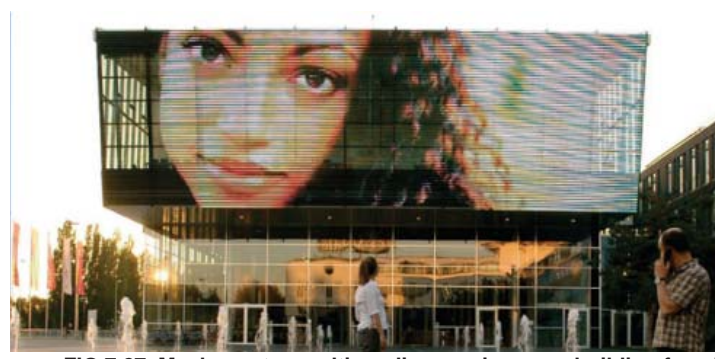
FIG 7.27_Mesh creates multi-media experience on building facade
