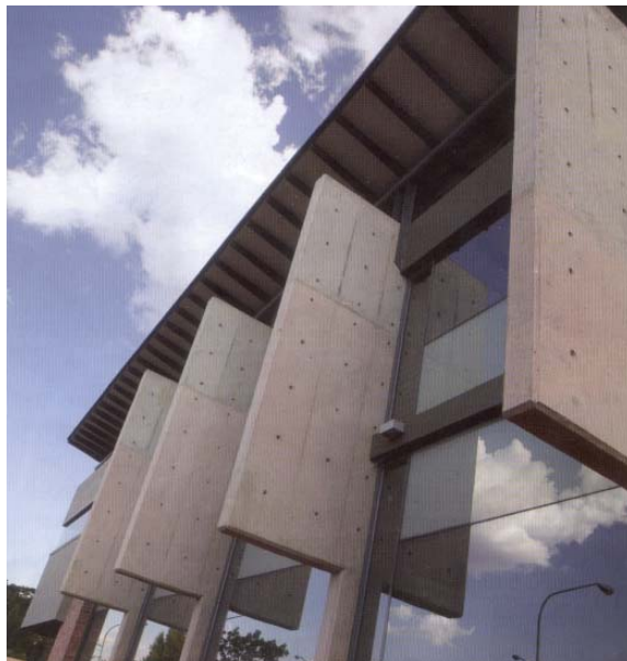
FIG 7.17_Off shutter concrete
