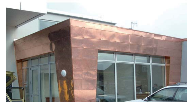
FIG 7.21_Newly installed copper cladding
