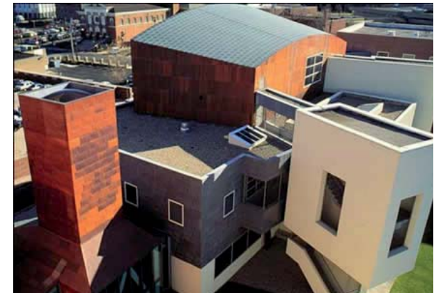
FIG 7.19_Weathered copper cladding
