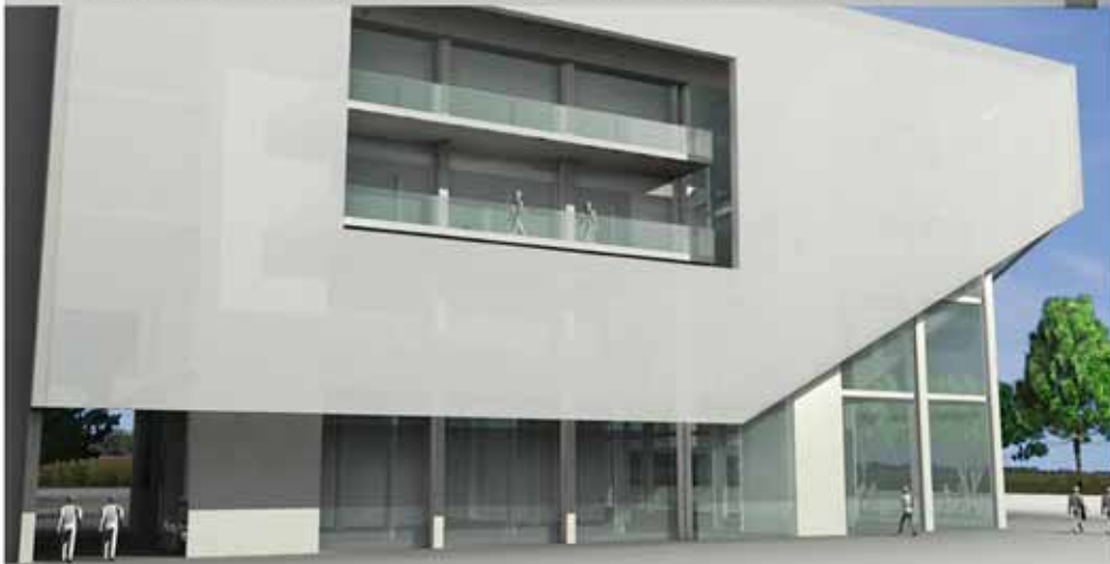
View of the northern facade of the building showing the pedestrian link to the east
