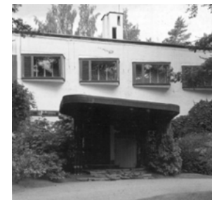
Fig 4.04 Entrance with climbing plants
