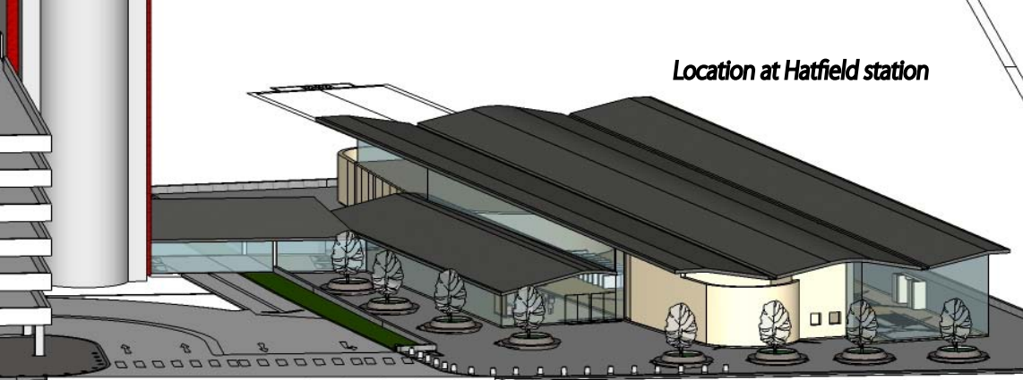
Hatfield station from the west (Grosvenor St.)
