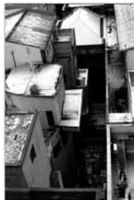
Fig. 36 Photos of Courtyard
