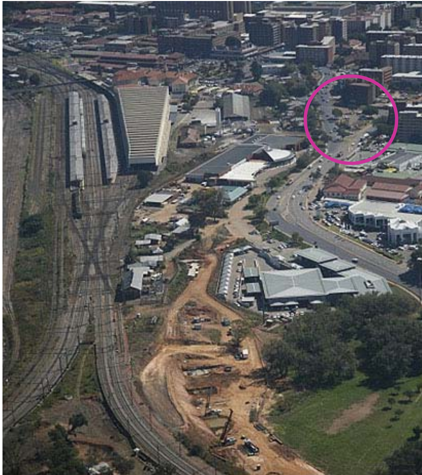
Figure 5-4: Aerial view of site (Source: Railways Africa, 2009)
