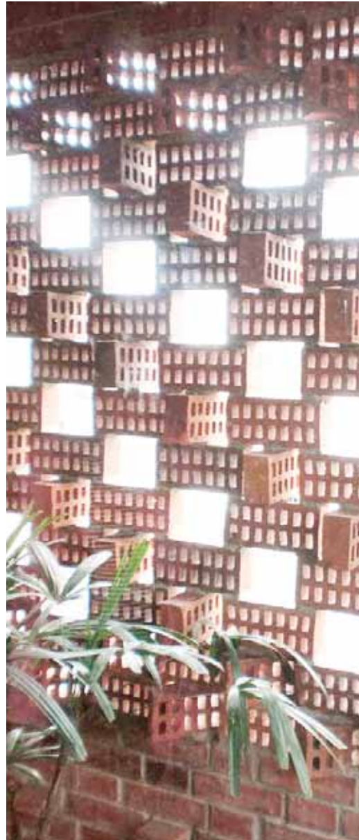
Figure 5.17: Woven face brick screens of the GMT Institute Of Property Management. (PLH Architects, 2012)
