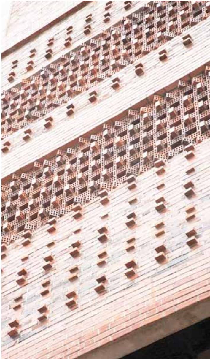
Figure 5.17: Woven face brick screens of the GMT Institute Of Property Management. (PLH Architects, 2012)
