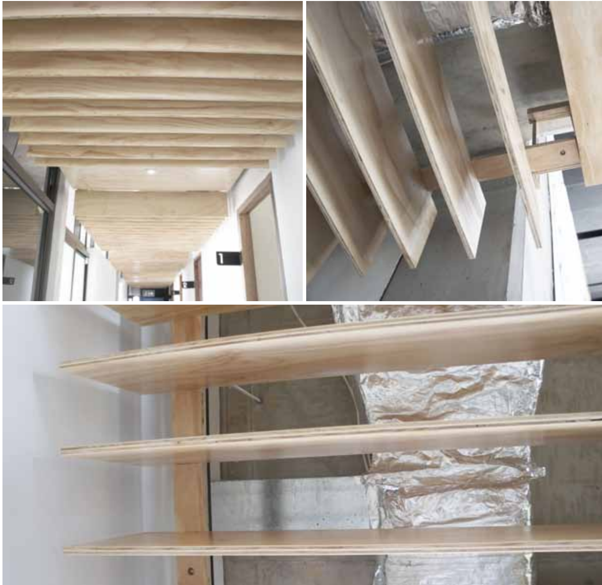
Figure 5.24: Photographs of the ceiling structure in the NoviSkin building. (Raubenheimer, 2012)
