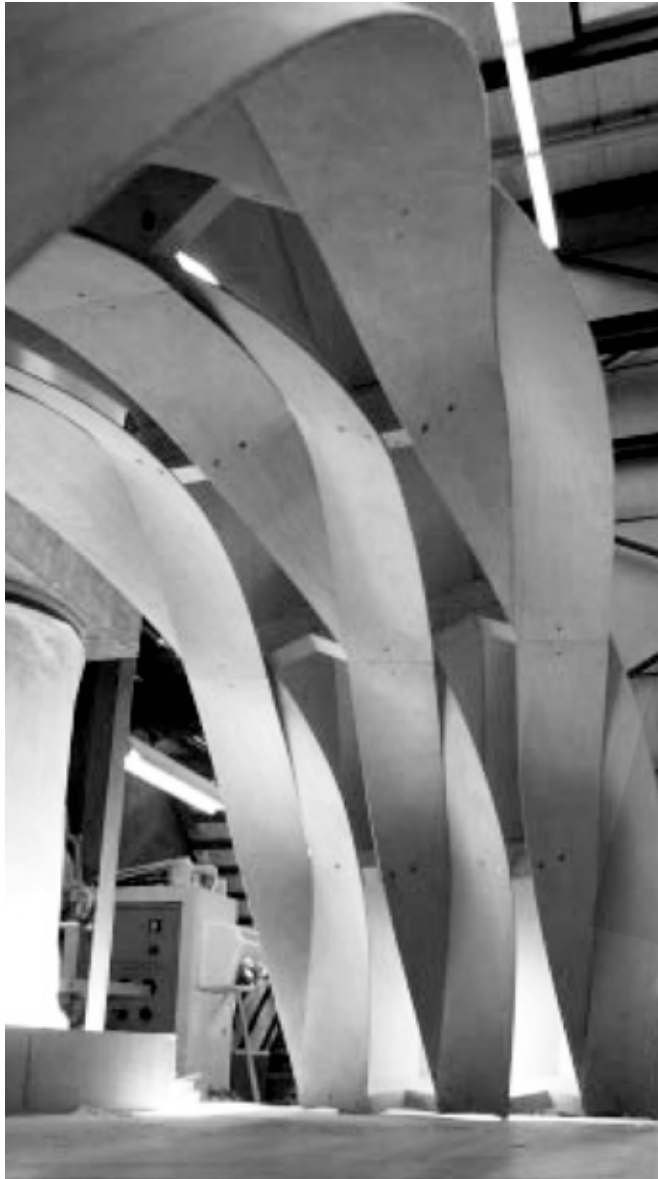
Figure 4.10: Braided structural timber arches from the Textile Module. (Hudert, 2010: 105)
