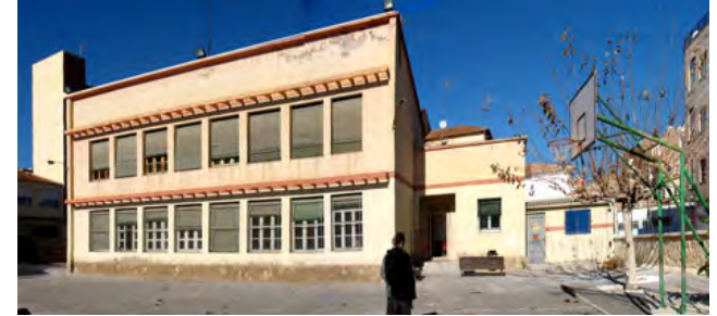
Fig.4.9 Existing school building that was converted
