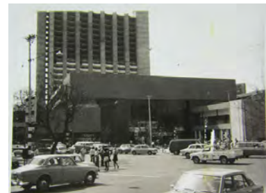
Sunnypark Mall under construction, 1974
