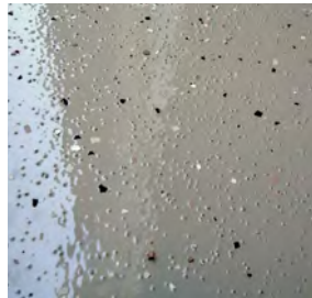
Fig.7.98 Detail view of epoxy flooring with grit
