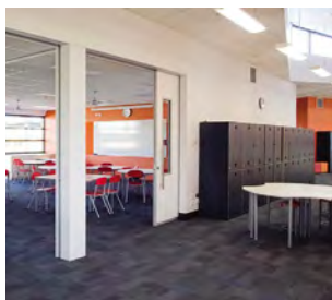
Fig.7.6 Acoustic sliding cavity door
