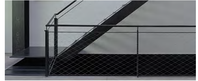
Fig.7.78 Staircase with ss wire rope mesh infill
