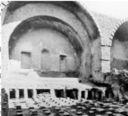
Figure 93. Photograph of the raised floor of the thrermae of Pompeii. showerman 356
