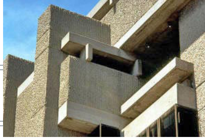
fig. 4.12 : Exposed concrete aggregate as finish to intersecting rectangles.
