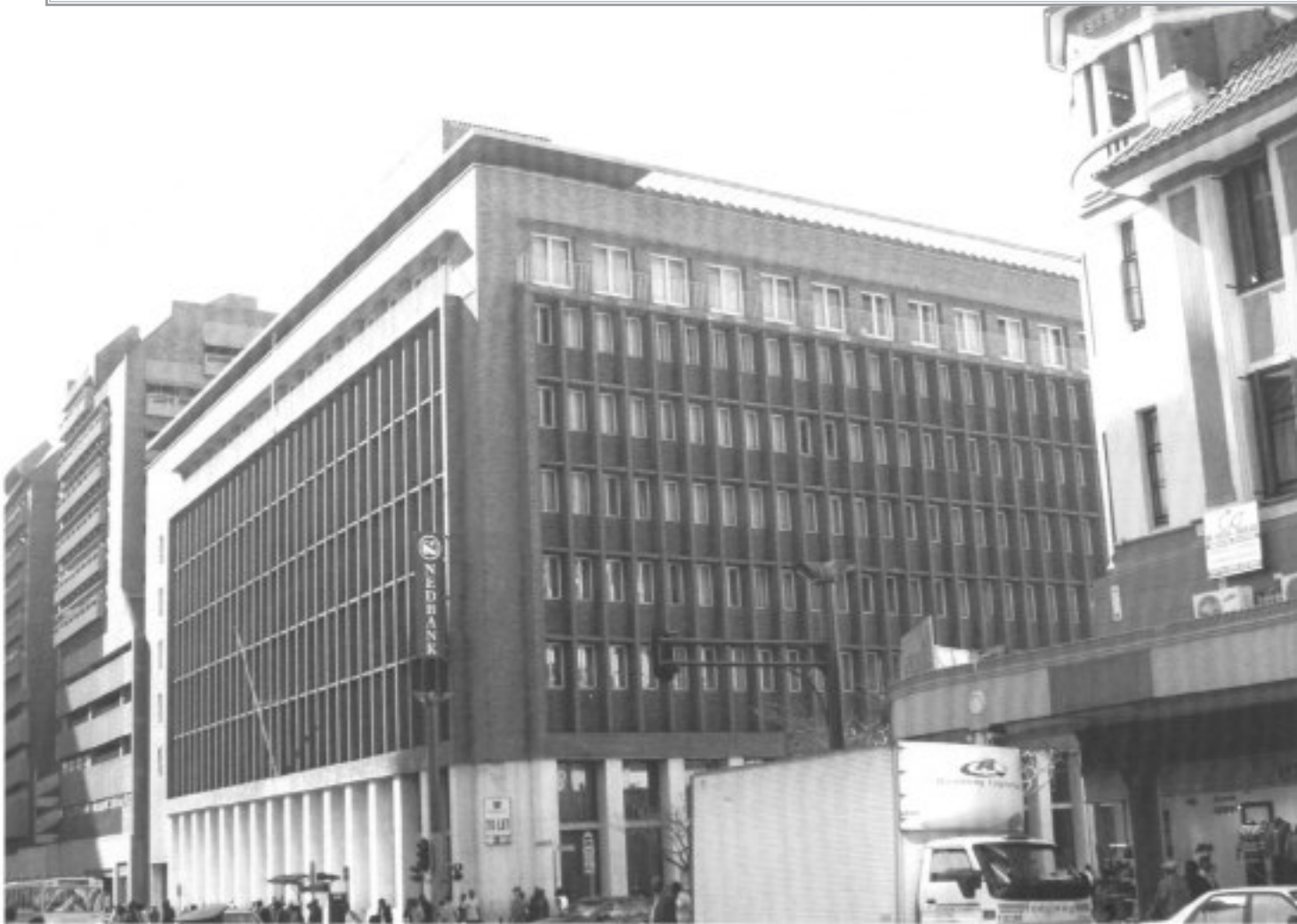
fig. 4.2 : The Netherlands Bank was designed in 1953 by Norman Eaton. The building was a summary of the Brazilian notions used in the Ministry of Transport building: vertical hardwood louvres on the west facade and a roof garden, inspired by the acclaimed Brazilian landscape architect Roberto Burle Marx. Eaton took great care in his projects to have the exterior spaces compliment the building.
