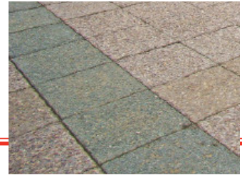
exposed aggregate concrete
