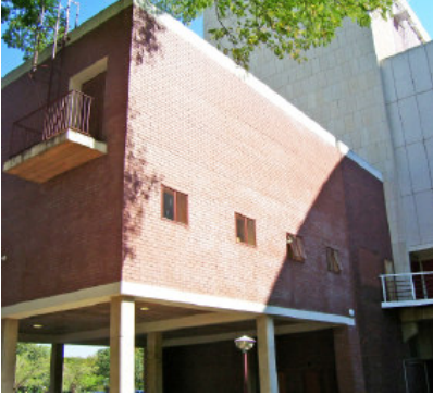
red brick, stucco & rough-hewn stone
