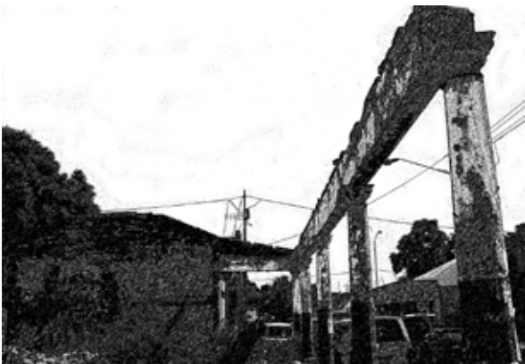
Figure 5.1 Partly demolished structure in Grand Street (Author, 2010).
