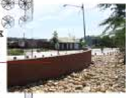
Figure 6.3.g View from Jazz Park. See existing structures of IBR-sheeting and face brick (Author, 2010).
