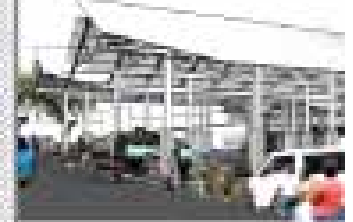
Figure 6.3.f Proposed Recycling Centre. Notice portal frame structures (Kunz, 2007).
