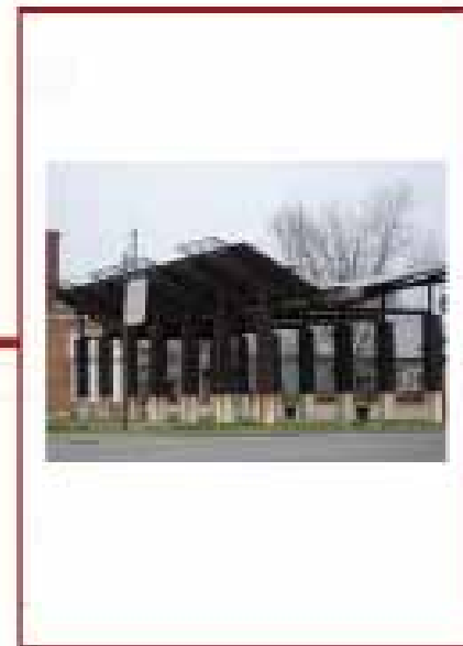
Figure 4.18 Columns with bulky appearance and roof with light aesthetic (Oppenheimer, 2002:134).
