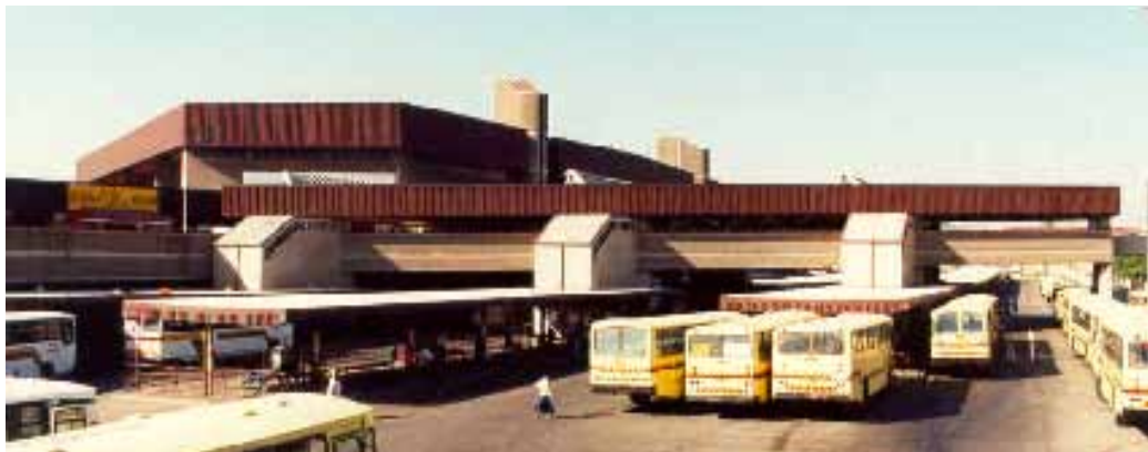
Figure 2.14 Belle Ombre Station, important transport node in Marabastad. This building has the largest scale in the area (Tayob, 2005 : 190).
