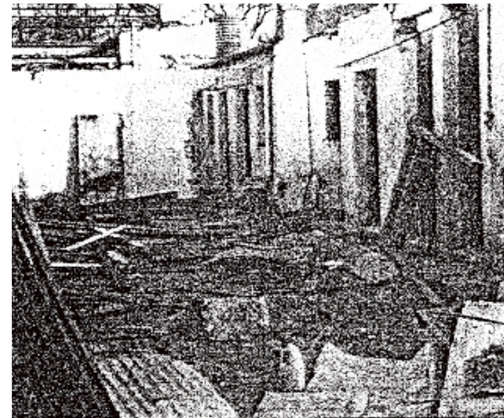
Figure 2.9 Demolition of 377 Cowie Street during 1972 evictions (Holm Jordaan & Partners, 1998).
