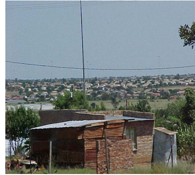
Figure 2.8 Extended room with corrugated roof sheeting illustrating typical township extension principles.
