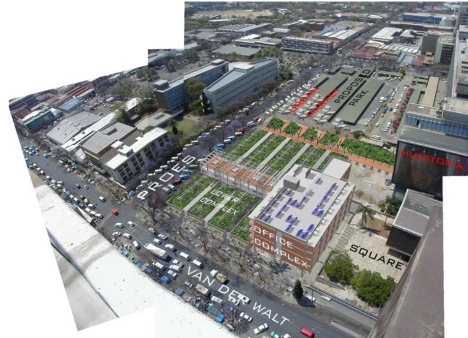
Fig 19: Aerial view of project
