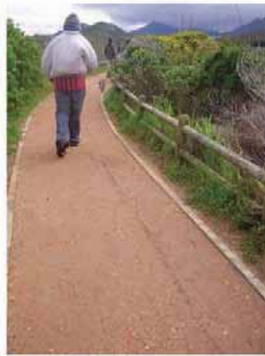
Soilcrete paving (Author, 2008)
