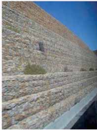
Gabion wall (Author, 2007)
