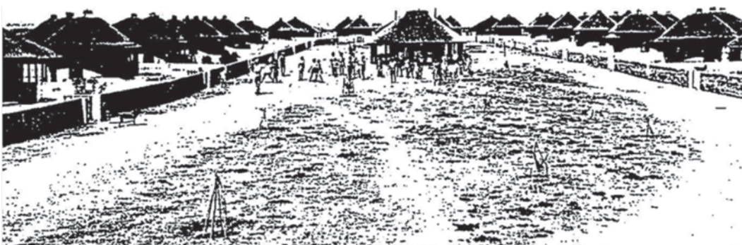
Figure 8: The first housing in Mamelodi showing lapa system (Walker & Van Der Waal, 1991)
