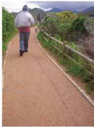
Soilcrete paving (Author, 2008)
