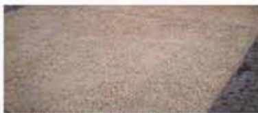
Exposed aggregate concrete paving (Author, 2007)
