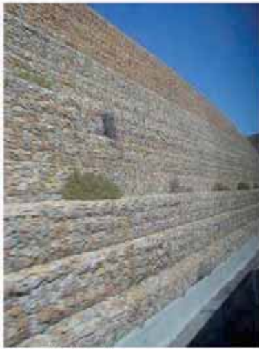
Gabion wall (Author, 2007)
