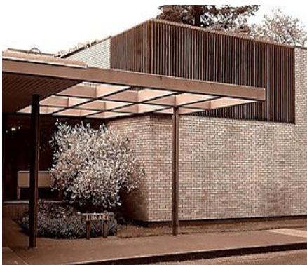
illus. 5.6a Brick exterior
