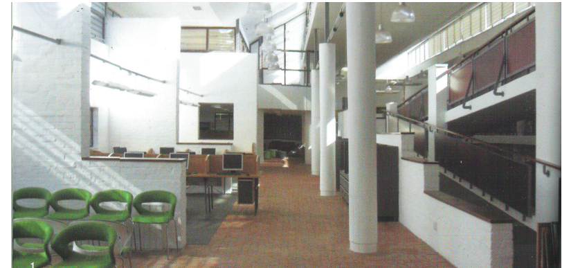
illus. 5.17 Main circulation space with brick paving, and natural lighting from saw-tooth roof clere storey windows
