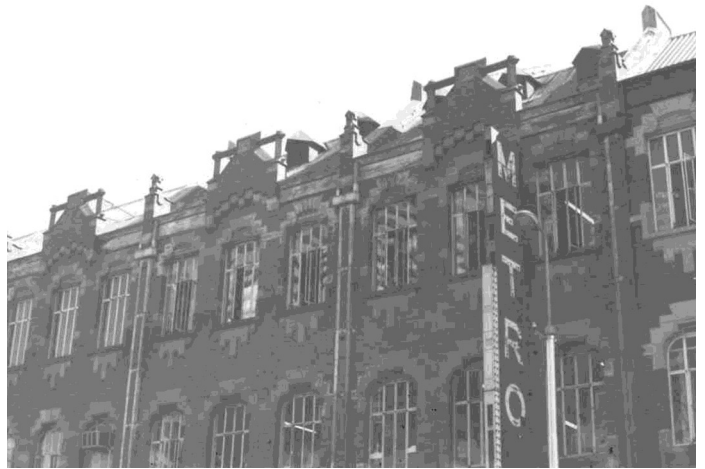
A3.11. Photograph of Lewis & Marks building: South elevation
