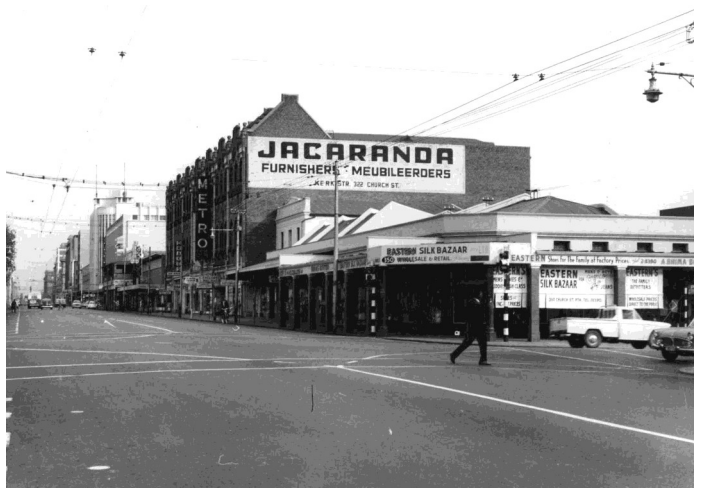
A3.15. Photograph of Lewis & Marks building: context
