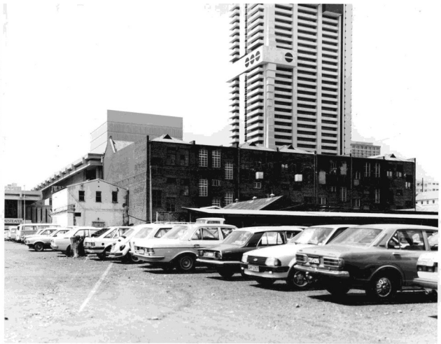
A3.12. Photograph of Lewis & Marks building: North elevation
