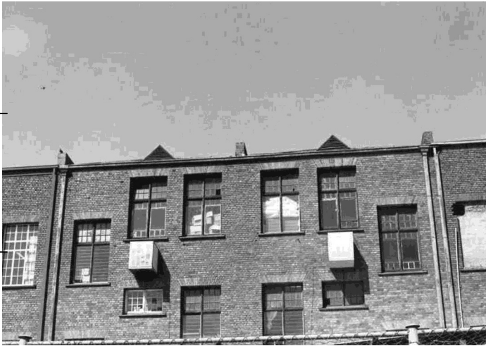
A3.10. Photograph of Lewis & Marks building: North elevation
