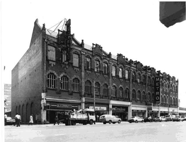
A3.14. Photograph of Lewis & Marks building: South elevation
