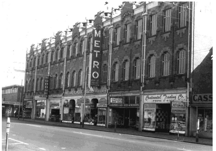
A3.13. Photograph of Lewis & Marks building: South elevation
