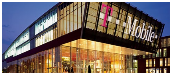
Illus 8.33. Media-mesh on a building.
