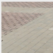
Illus 8.38. Sammy Marks Square: Concrete paving, natural and pigmented. Good condition.
