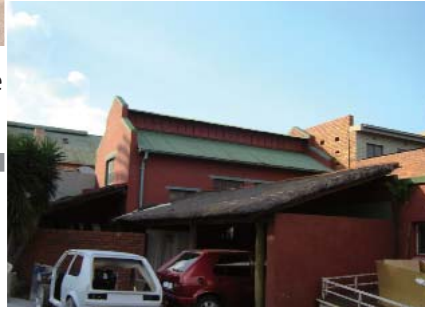
Figure 7.3.14 Photo of character of the existing building to be retained (Author, 2011).
