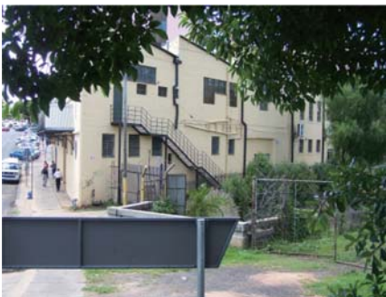
Figure 7.5.21. Building adjacent to Walkerspruit (Author,2011). The building in the background fronts Pretorius street and the western facade fronts onto Walkerspruit and Caledonian. The building is currently occupied by a church and Christian book store.
