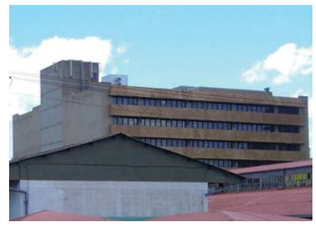
Figure 7.5.26. Benstra building (Author,2011). The south and western facades of this multi storey building defines the project site. The buildings northern facade create a strong urban edge onto church street but offers no pedestrian interface with the street.
