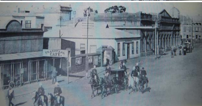
Figure 7.2.15 Photograph of Church Street at the time (Andrews, 1989).
