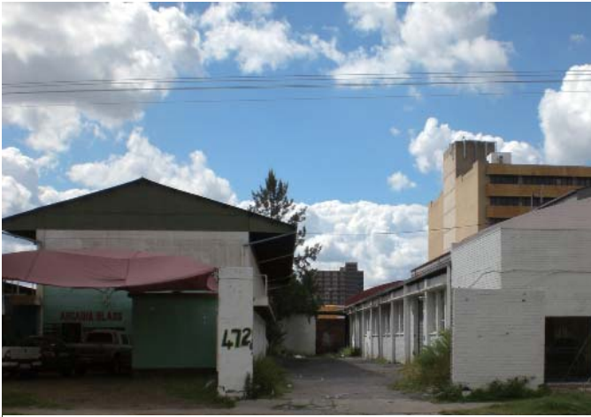
Figure 7.3.18 Existing industrial buildings on site to be retained (Author, 2011).
