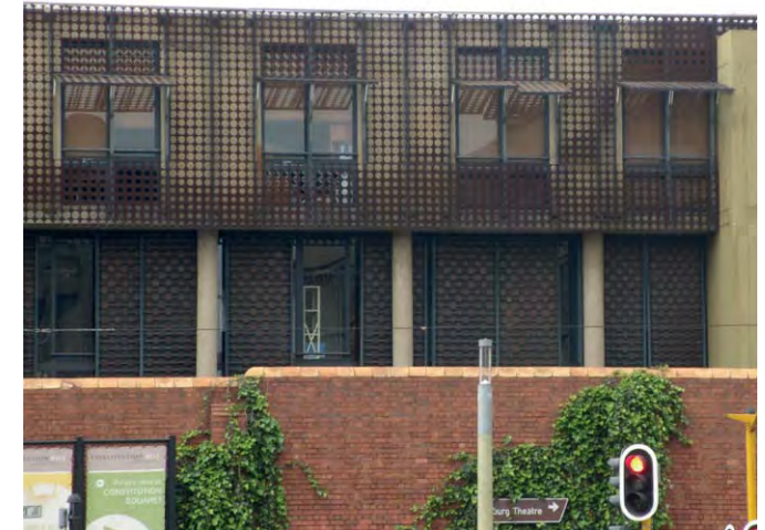
Fig. 7.37. Kate Otten's Women's Jail Precinct - the Cor-ten screens (Author, 2011).
