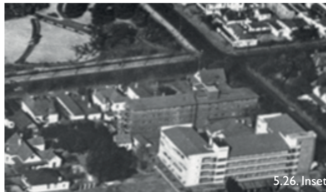
Fig. 5.26. Aerial photo of Pretoria in 1949. Inset: zoomed image of the selected site reveals the Park Lodge building, the Transvaal Pyramid Roof house and a house on the proposed site for the dissertation. (Pretoriana Archive Collection, Department of Architecture, University of Pretoria, 2011).
