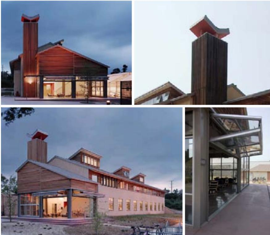
Fig 5.22: Views of roof openings for maximum daylight exposure (Carboun 2010)
