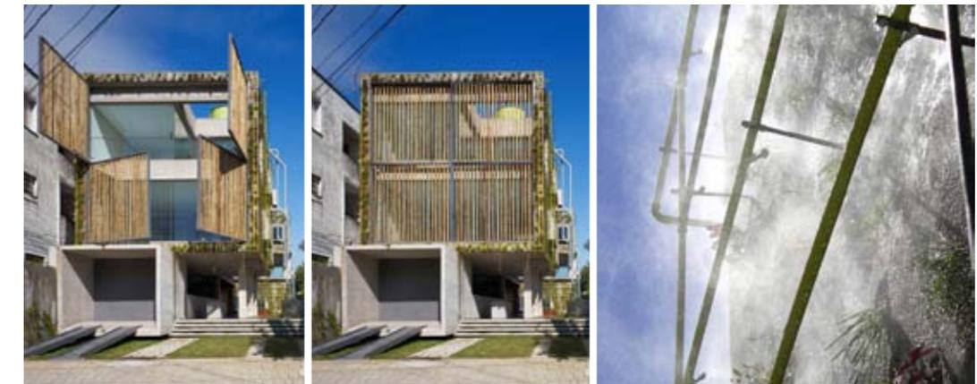
Fig 5.20: Irrigation system on façade (Triptyque 2008)
