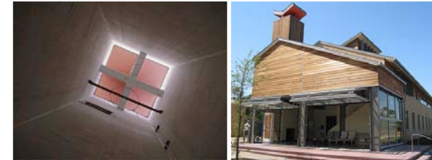
Fig 5.29: Views of the building's cooling tower [Carboun 2010]
