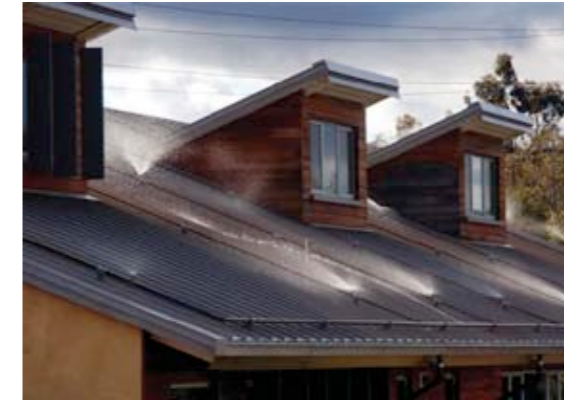
Fig 5.22: Views of roof openings for maximum daylight exposure (Carboun 2010)
