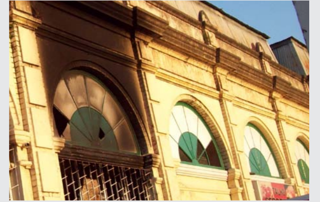
Illus. 134: Fire Damage, historic market building, Baixa (author, photo June 2011)
