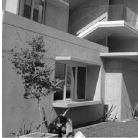
Off-shutter finish according to grid with exposed tie
