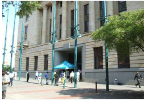
Illus. 2.2: The architectural language of the First National Bank in Church street, Pretoria, could to be perceived as a stronghold of power, strength and safety, but can also be imposing. (Author, January 2006)
