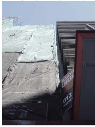
2.18 PRESIDENT TOWER. FACADE
