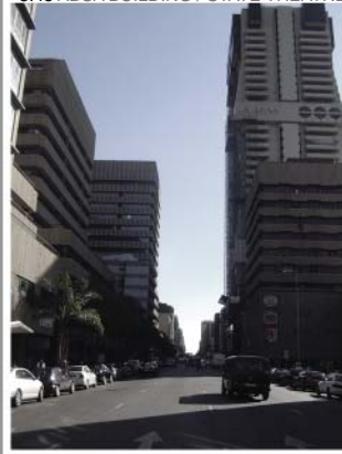
3.45 ABSA BUILDING / STATE THEATRE
