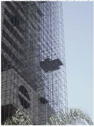
2.17 ABSA BUILDING. RENOVATION
