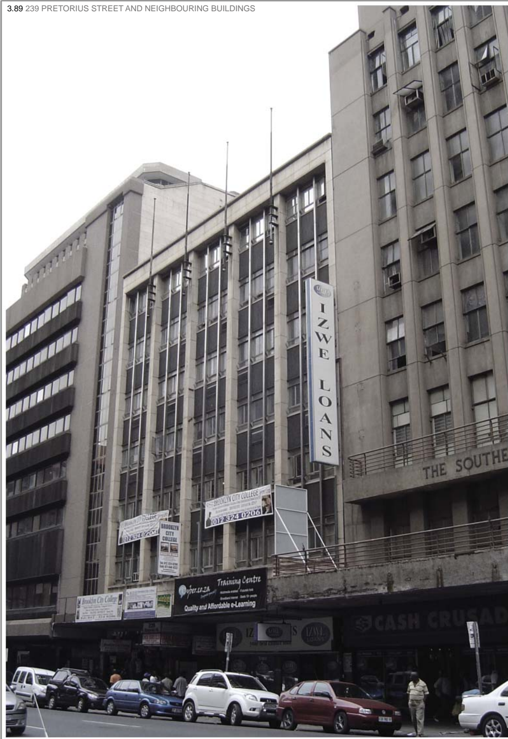
3.89 239 PRETORIUS STREET AND NEIGHBOURING BUILDINGS
