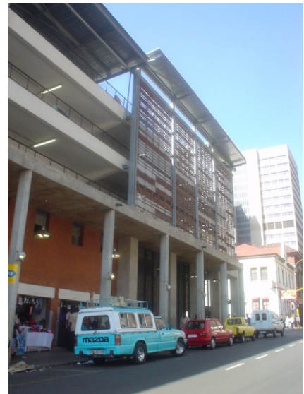
Figure 39. Use of Materials in Newtown
