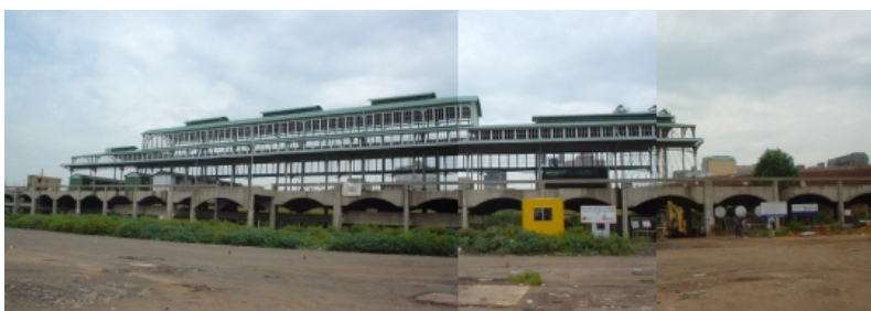
Figure 21. Old Parktown Station
