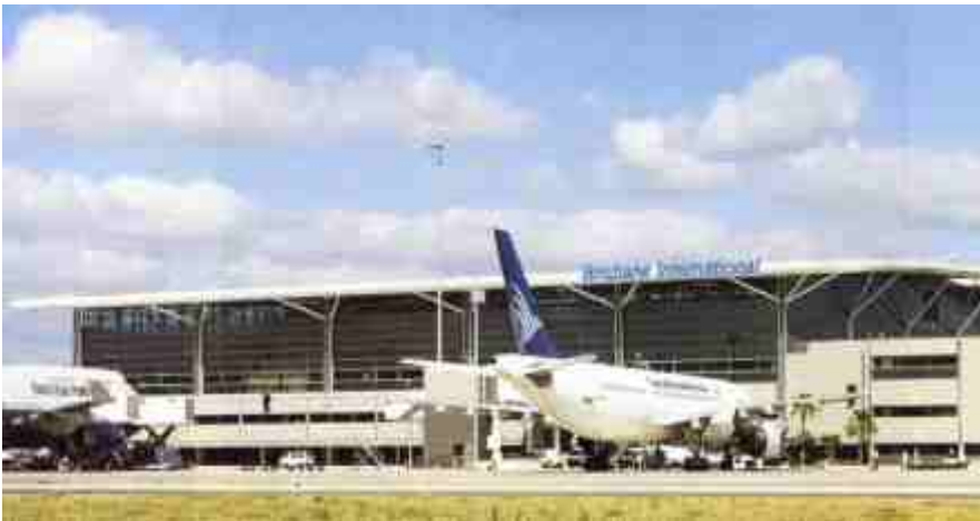
Figure 5.5.3. Above The Terminal Building by day(World Architecture July/August 1996:129)
