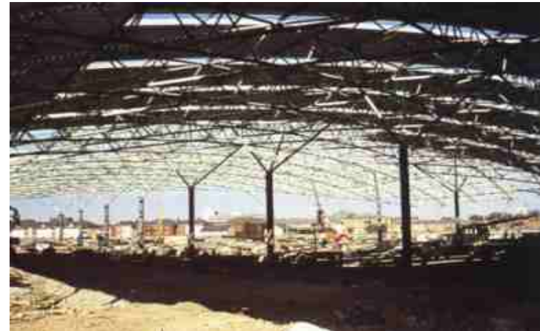
Figure 6.3 The design of the canopy in the Gautrain Station, Hatfield will be similar to the canopy at Stratford Market Maintenance Depot. Note the use of rooflights. (World Architecture April1996;110)
