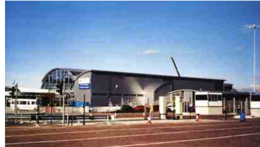
Figure 6.1 The Holyhead Ferry Terminal Building. The use of modular building methods inspired the curved roof shape in the design of the Gautrain Station. The ease of add-on in the building process would make it possible for the Station to be cost-effective. (World Architecture July/August 1996:126)
