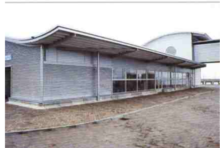
Figure 6.2. Holyhead Ferry Terminal Modular Roofing Construction. (World Architecture July/August 1996:126)
