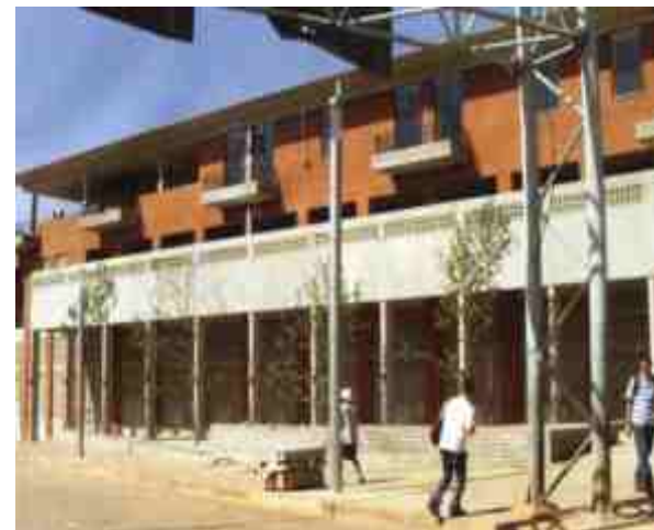
figure 5.2.5 West street facade,Metro Mall ,Newton, Johannesburg.(Leading Architecture:41)
