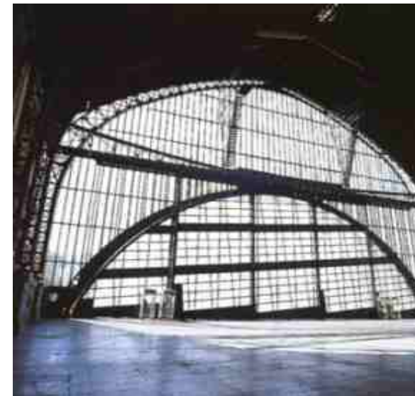
figure 5.3.3. Interior showing the new glass doors.(World Architecture July/August 1996:57)
