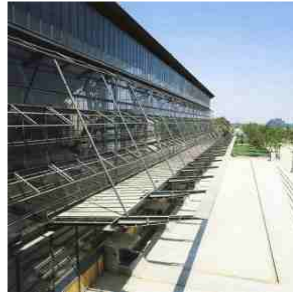
figure 5.3.2. The glass river façade with louvred wall to control heating.(World Architecture July/August 1996:57)
