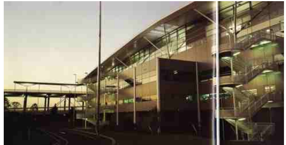
figure 5.5.1. Above View of the full height glazed walls and white colorbond roof. (World Architecture July/August 1996:128)
