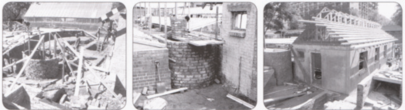
Figure 69: The Greenhouse Project construction photos.
