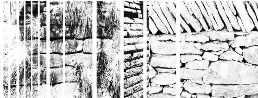
NEW LOOSE PACKED NATURAL RECLAIMED STONE RETAINING WALLS
