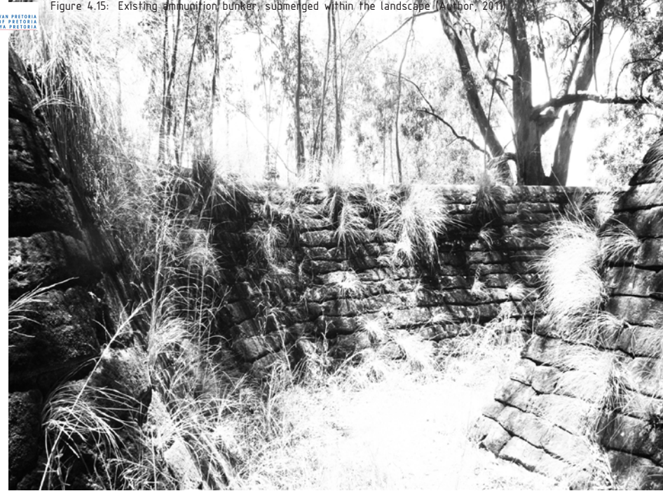
Figure 4.15: Existing ammunition bunker submerged within the landscape (Author, 2011)
