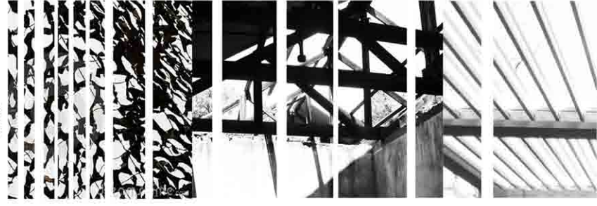
ROOF TRUSSES AND MILITARY SHADING DEVICES
