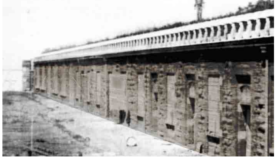
Figure 2.8: Central magazine during construction, 1984 (SANMMH)
