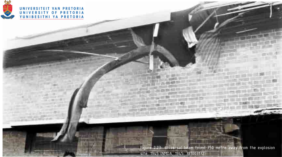
Figure 2.24: Bent structural member of the Grand Magazine found on site, 1945 (NMDA, 1945: 781003166)
