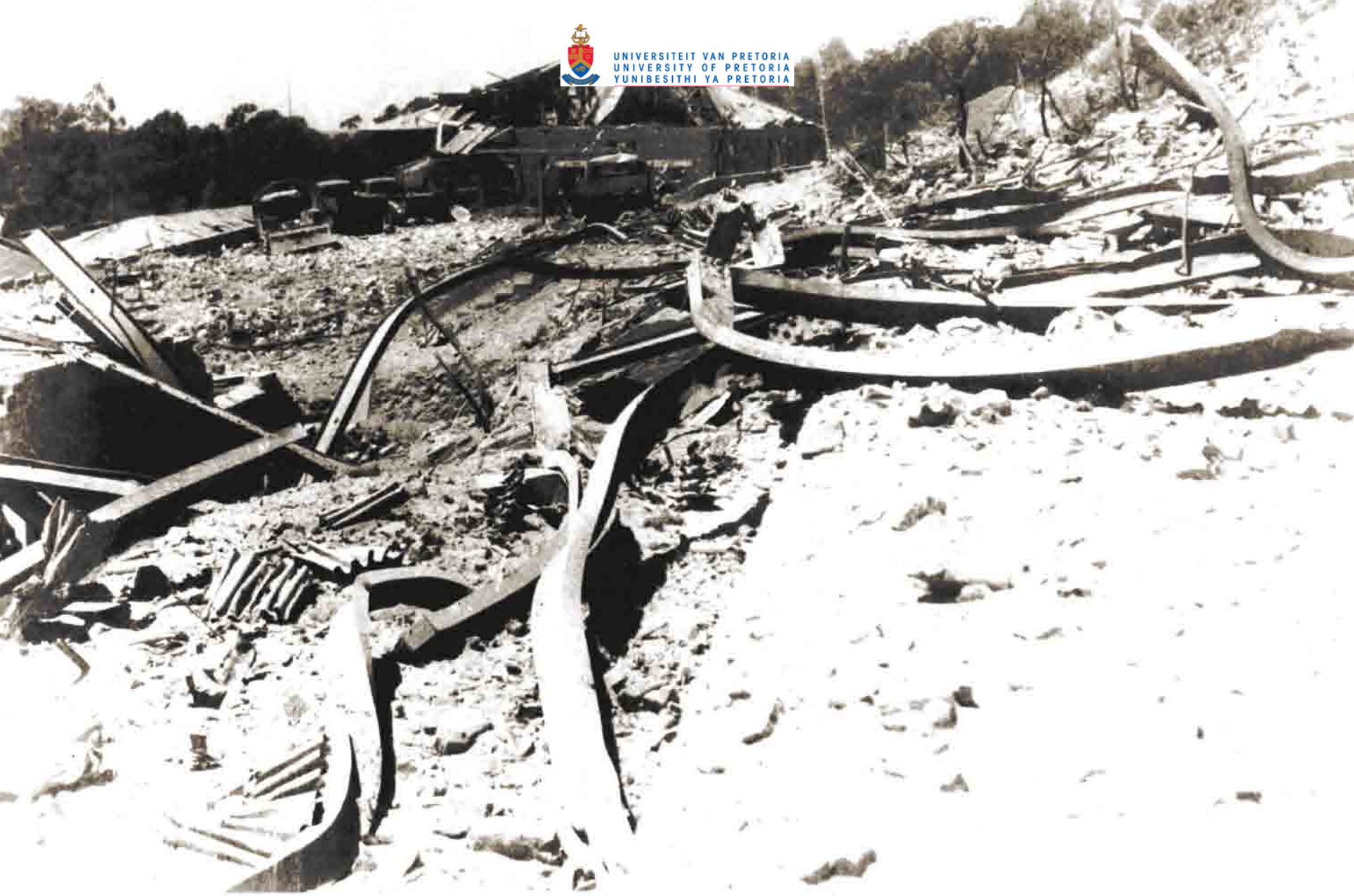
Figure 2.16: Magazine Hill after the explosion, 1 March 1945 (NMDA, 1945: 781003142)
