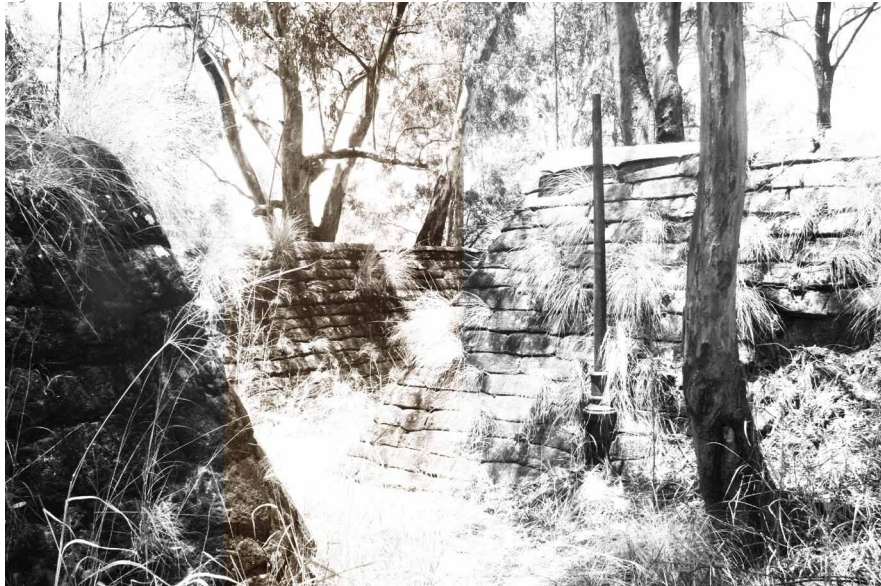
Figure 1.6: Interior view of submerged bunker space on Magazine Hill (Author, 2010)
