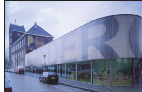
fig.7.33. Bredero School Building
