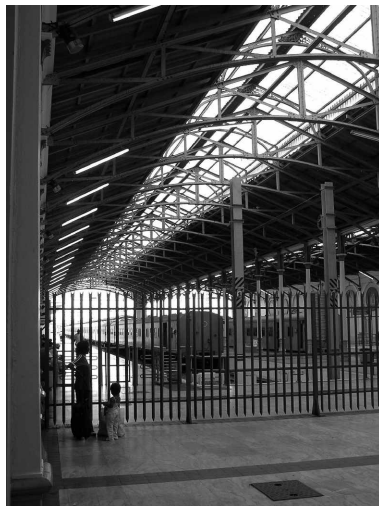
Figure 19. Interior perspective of the waiting area of the Station. Access to the perron can only be gained via a gate through a 'cheap and nasty' palisade fence made of devil's fork steel sections. These 'temporary measures' detract from what could be a pleasant experience
