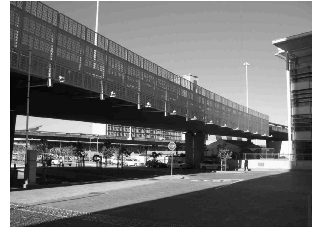
Figure 000. Sound baffles against the edges of the N2 highway that passes through the central courtyard of the CTICC.
