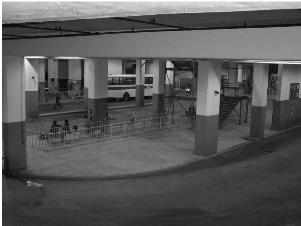
Figure 23. Interior view of the Algoa Bus Station.
