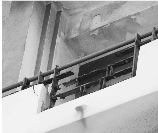
Figure 27. This beautiful Art-Deco balcony have just about rusted and blistered away.
