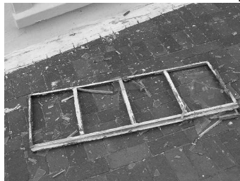
Figure 28. A complete window casing came loose during a brief spell of gusts
