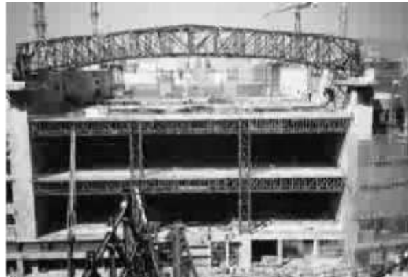
Six 280-tonne primary steel trusses were fabricated off-site. Secondary trusses were erected between the primary trusses to stabilise the roof frame and support the purlins for the roof deck.
