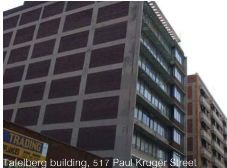
Tafelberg building, 517 Paul Kruger Street Fig. 5.6: Masonry and exposed structure
