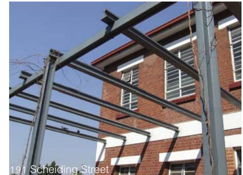
191 Scheiding Street Fig. 5.3: Railway line steel pergola
