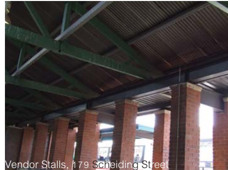
Vendor Stalls, 179 Scheiding Street Fig. 5.12: Sheet metal roof + exposed timber truss
