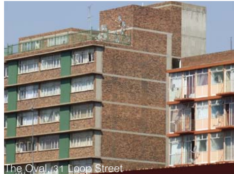
The Oval, 31 Loop Street Fig. 5.9: Masonry and exposed structure
