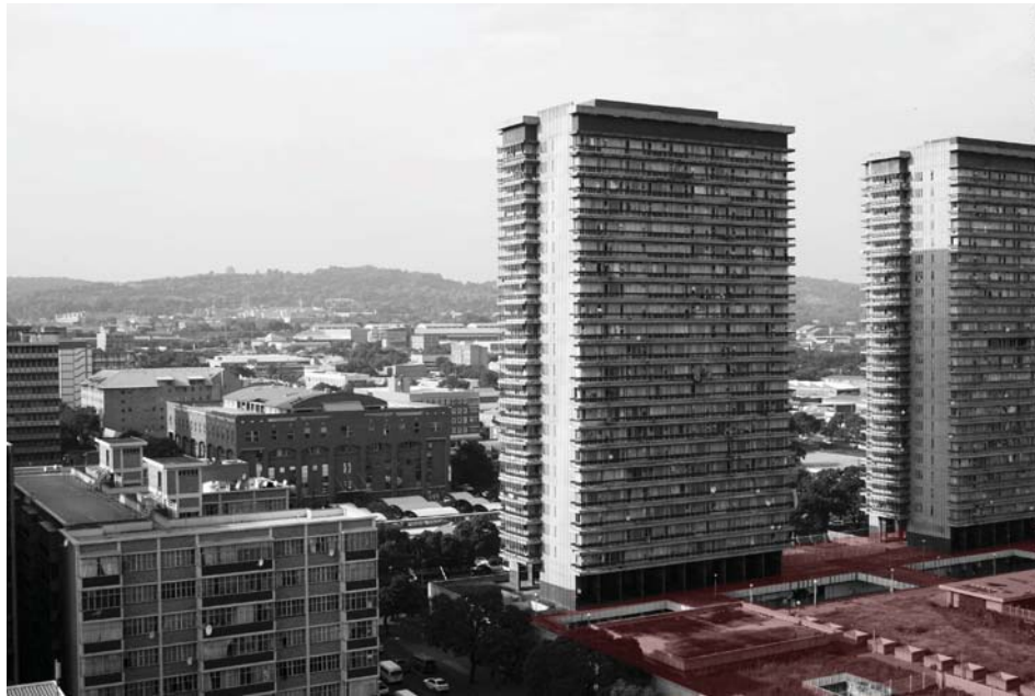
Fig. 3.25: Schubart Park illustrating residential blocks and courtyard
