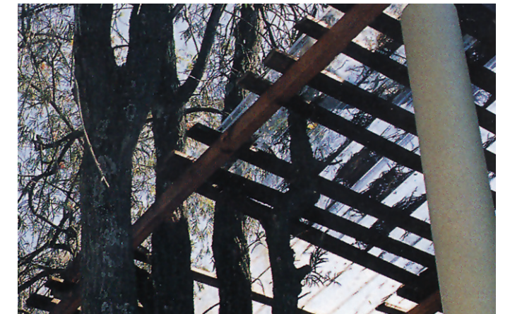
Fig. 5.3.5 Lightweight pergola structure
