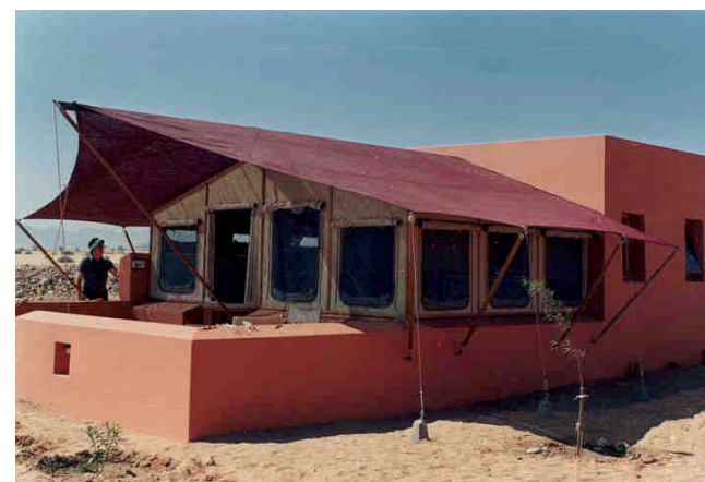
Fig. 5.4.5 North-western view with higher eastern wall
