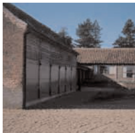
Fig. 5.1.4 Shaded southern facade
