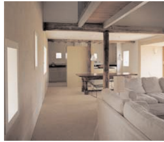
Fig. 5.1.3 Timber structural columns
