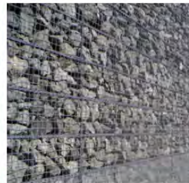
fig 162. Gabion walls. (Google images)
