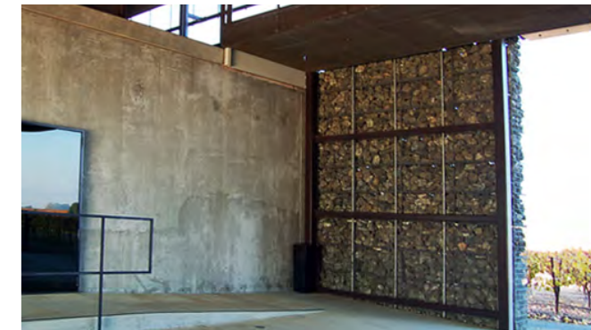
fig 149 b. Interior view of Winery. ( MYD studio 2010)
