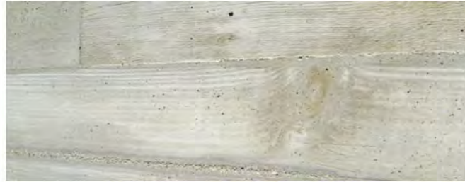
fig 163. Rough sawn off-shuttering. (Google images 2012).
