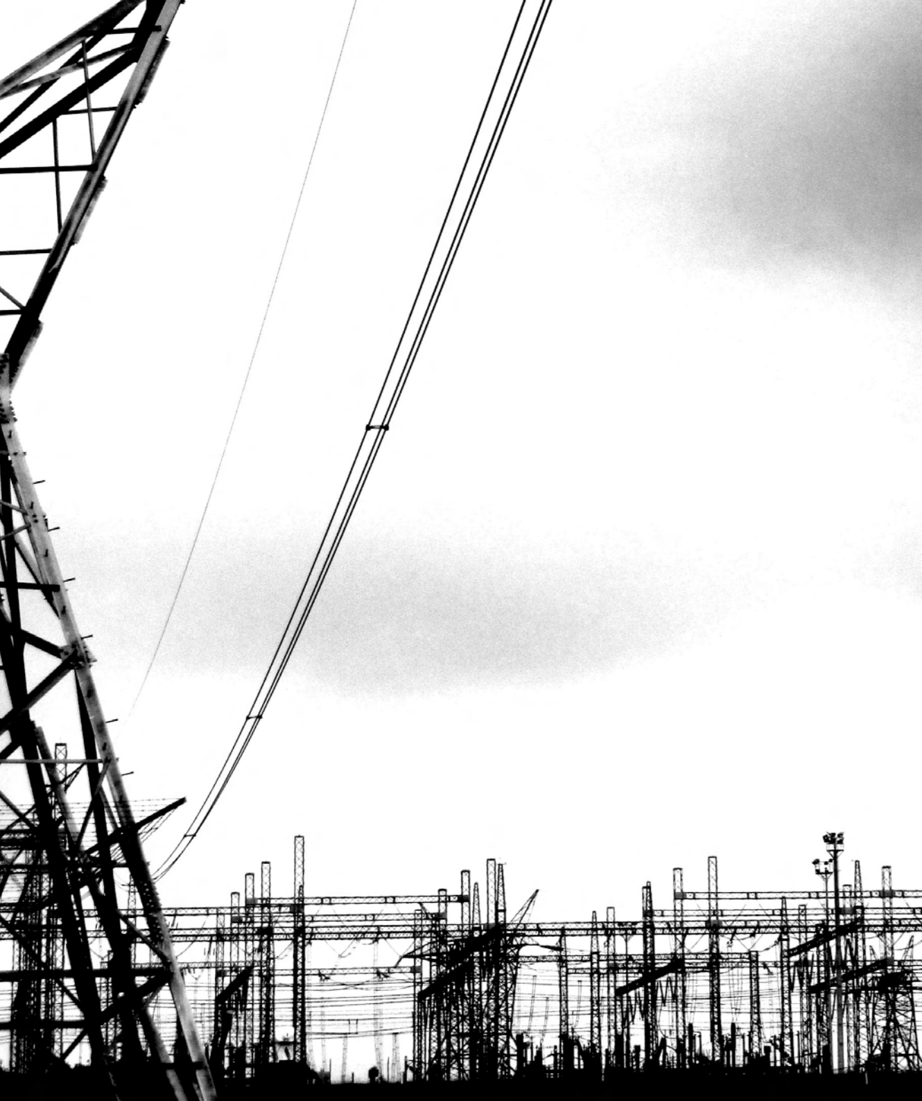
fig 12. Eskom power lines.
