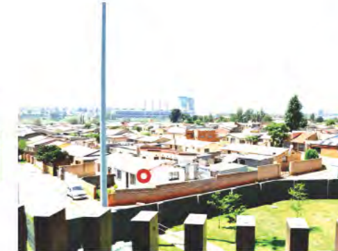
fig 24 d. Urban condition
