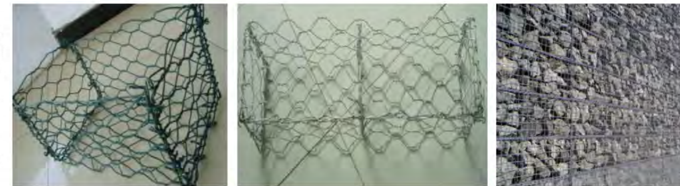
fig 162. Gabion walls. (Google images)
