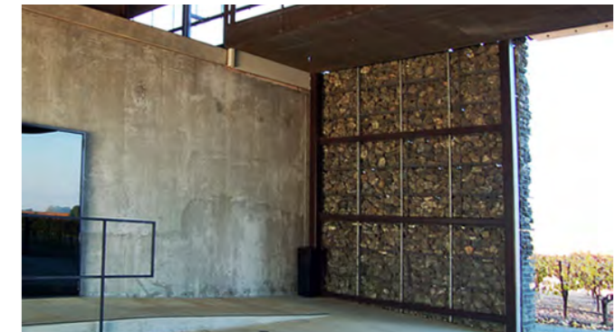
fig 149 b. Interior view of Winery. ( MYD studio 2010)
