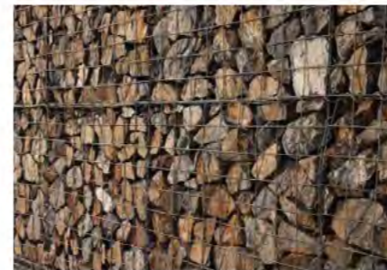
fig 160. Gabion wall (Google images)
