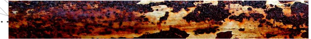
fig 89 g_. Rust and paint.
