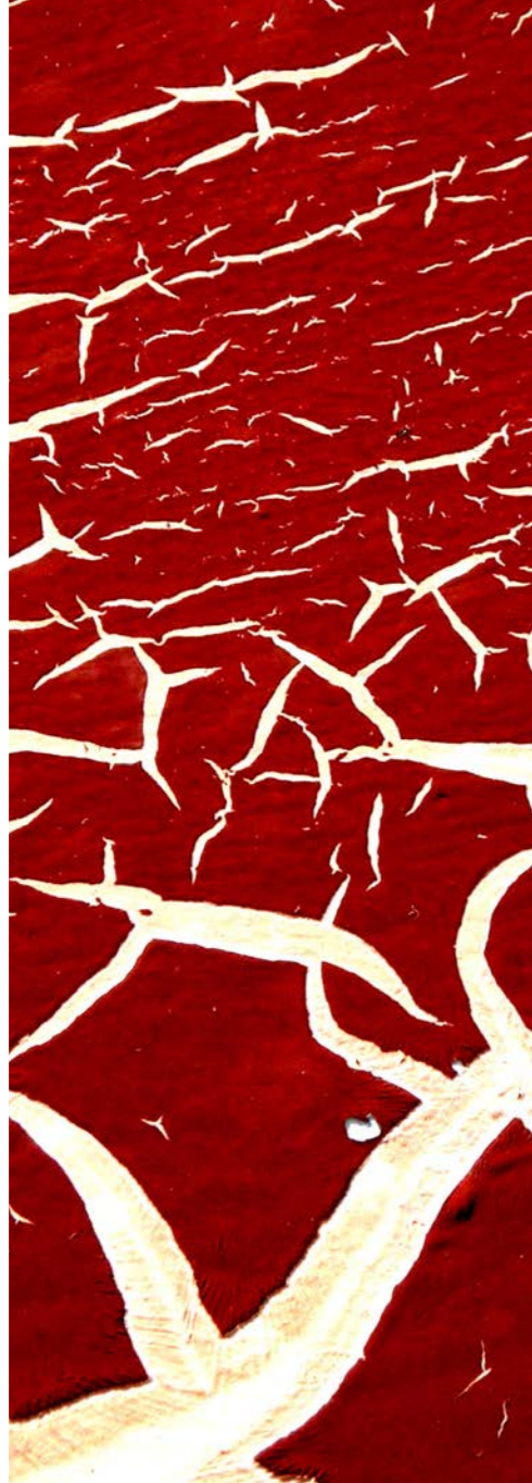
fig 97 b. Cracking paint.
