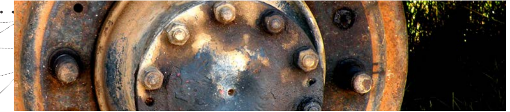
fig 89 a_. Rusted wheel.
