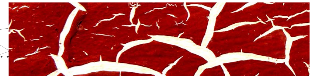
fig 89 d_. Paint flaking.
