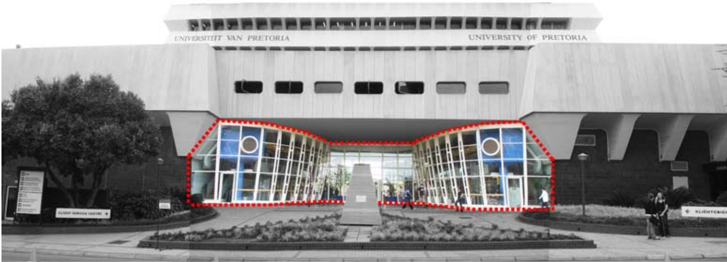
Client Service Centre
