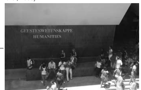
Fig. 3.25 Main entrance to Humanities building [Author, 2008]
