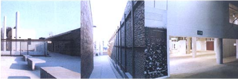
Figure 076: Various internal views
