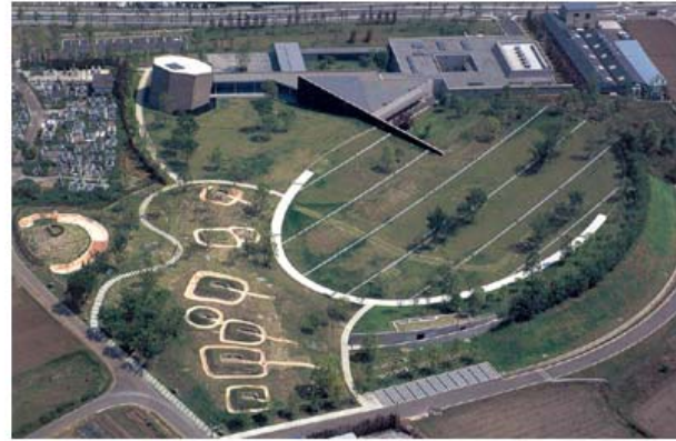
Figure 088: Aerial View of the Complex
