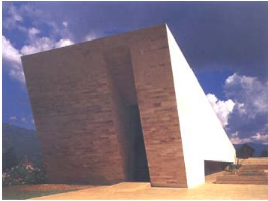
Figure 080: Main Entrance to Crematorium
