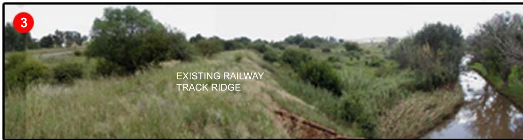
Figure 064: View Looking North
