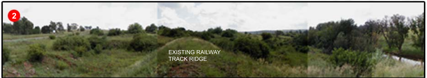
Figure 063: View Looking North
