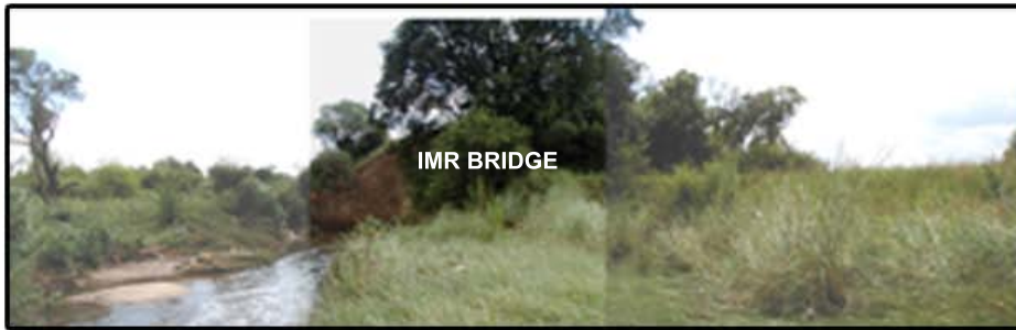
Figure 055: IMR Bridge - West Elevation
